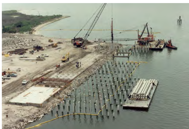
Pile driving operations in the Port of Tampa, Florida, United States.
