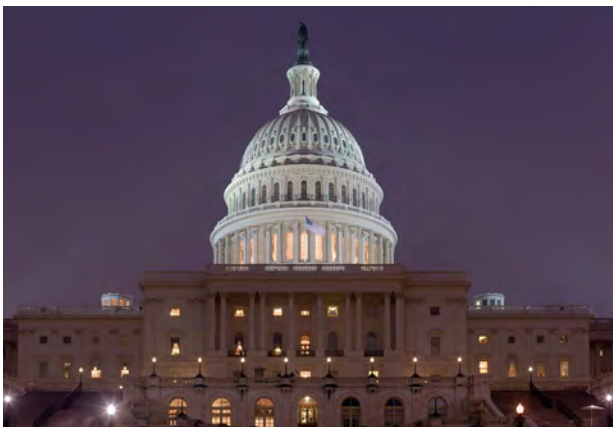
US Capitol Building.
